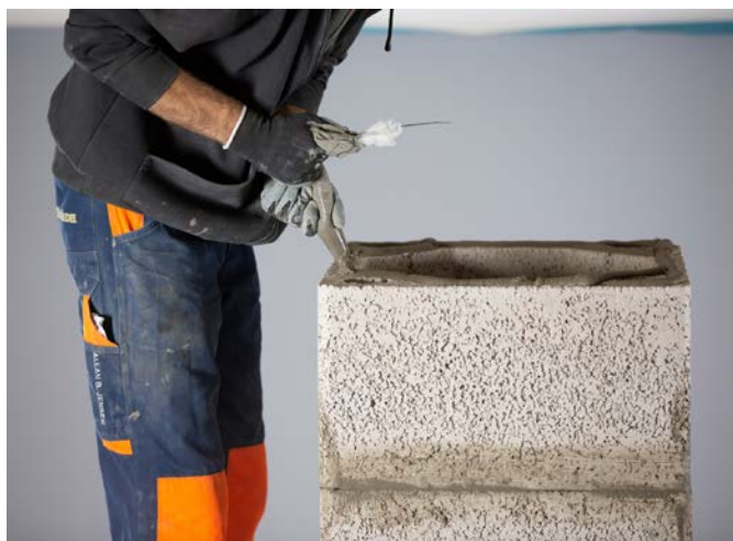
Glue on the next two chimney blocks.
