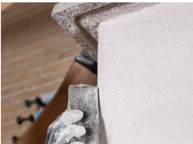
Ensure the edges are smooth and wait to dry.
