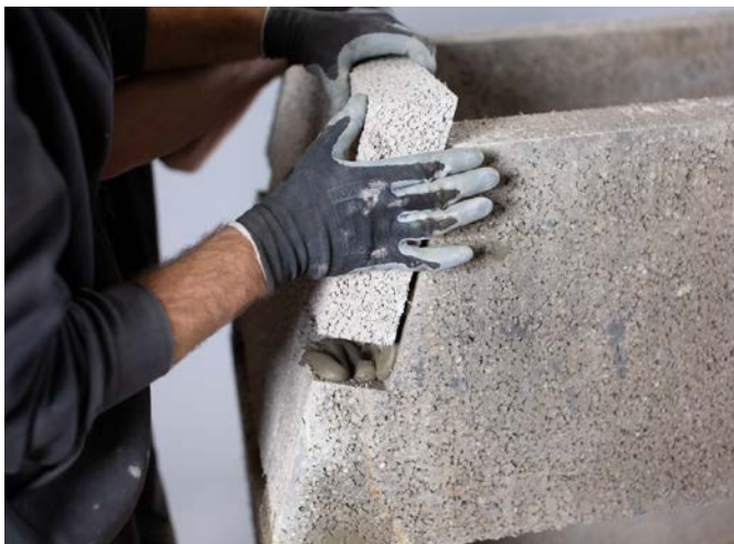
Press the side panels of the gather into place.
