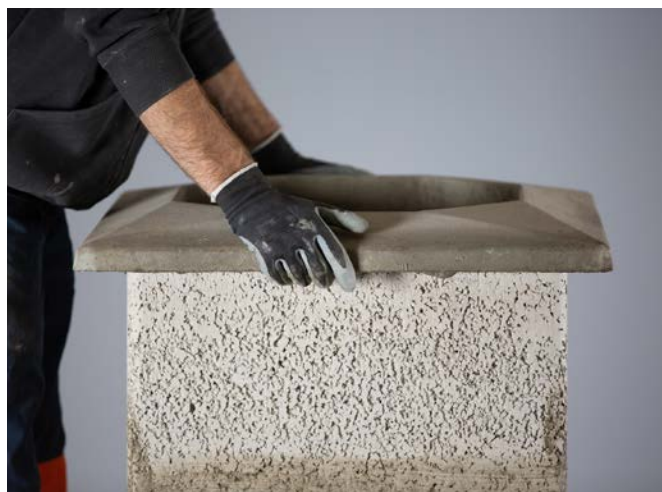
Glue on the capping.
