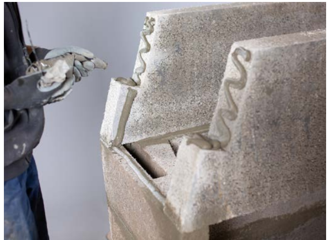
Apply lip glue to the joints on the sides of the front and rear panels of the gather.
