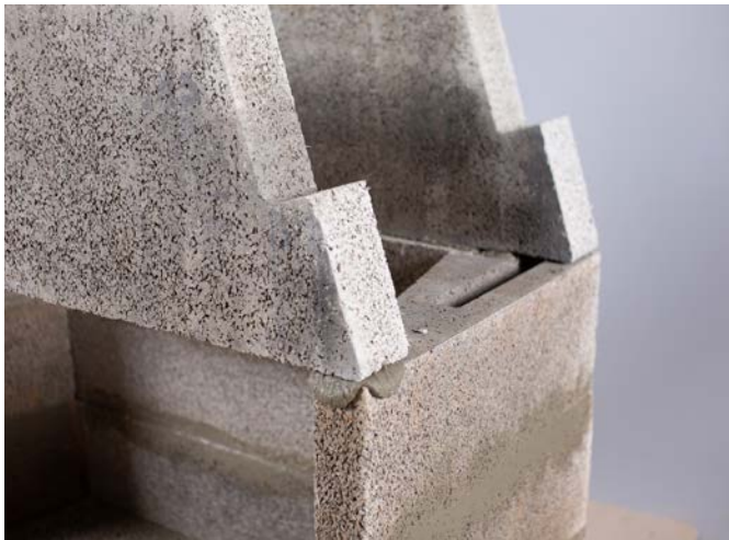
Apply lip glue to the top layer and then press the front and rear sections of the gather into place.
