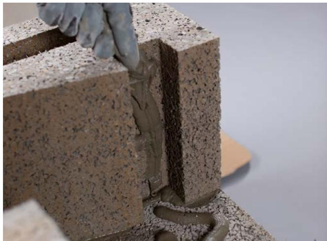
Press one side block into place and apply the lip glue into the slot as shown.
