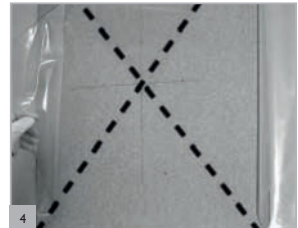
4 Cut a cross shape in the vapour barrier to the required dimensions of the opening (see figs. 1. and 2.)
