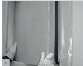
6 Remove wood fibre board, thermal insulation etc. from the assembly opening.
