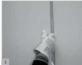
3 Remove plasterboard. NOTE: The vapour barrier must not be damaged!
