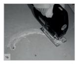
Cut a hole in the thermal board to fit the Ignis-Protect outer protection pipe. IMPORTANT: follow the safe working notes on page 31.
