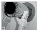
Example of a design with a double-walled connecting flue pipe.
