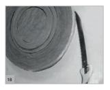
If necessary, shorten the inner and outer protection pipes to be flush with the wall. IMPORTANT: follow the safe working notes on page 31.
