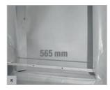
Check width of the opening: 565mm NOTE: Ignis-Protect must not be shortened on site!
