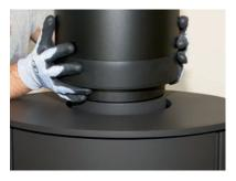
2. Place the concentric adapter and push the protruding liner onto the stove connector. If necessary, the adapter can be cut at the bottom to get the desired distance between the pipe and the stove top plate.
