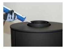
1. Make sure the concentric outlet on the stove is installed correctly, according to the installation manual for the stove. Apply high temperature liquid sealant on the inner and outer ring of the stove outlet to provide a gas tight connection.
