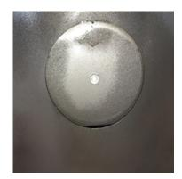
1.) Carefully remove the rear flue pipe cover plate by drilling out the tags next to each of the pilot holes (x6)
