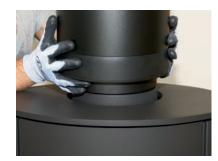
2. Place the adapter and push the protruding liner onto the stove connector. If necessary, the adapter can be cut at the bottom to get the desired distance between the pipe and the stove top plate.
