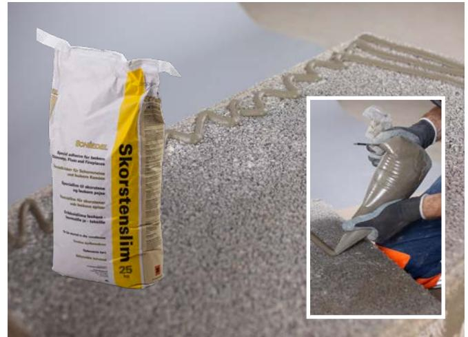
Mix lip glue jointing adhesive as per instructions on the bag. Apply 15-20mm beads using the supplied application bag as shown in the picture above.
