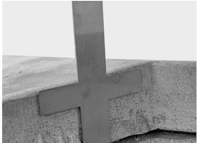
When the capping is being glued into place, slide the wave legs into the lip glue joint (as per pic).
