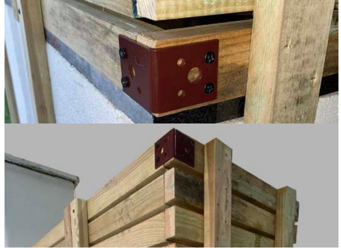
Attach the top and bottom metal brackets to the side and back panels.
