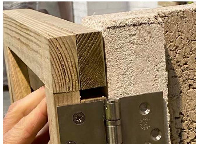
After rendering, align the hinge to the logstore, ensuring the door is below the top of the logstore (a 5mm gap is fine).
