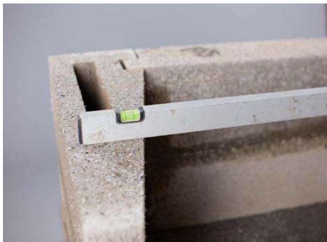
Add a further 2 layers of side blocks and back panels applying lip glue adhesive between each layer and at each joint. In total there are 3 layers on top of the base plate, as per the image. (If the log store option is not being used, then this base plate will be bedded directly on to a suitable prepared base.
