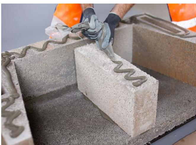
Press the middle section down on to the adhesive and apply additional adhesive as shown.
