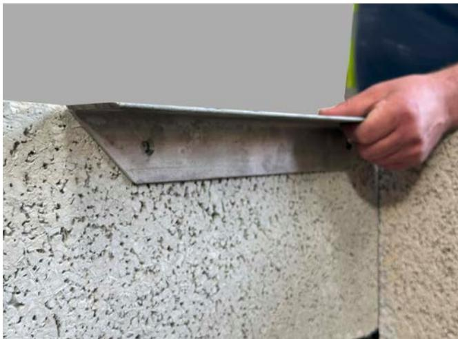
On both outer sides of the garden fireplace a metal bracket is to be fitted level with the top of the side stores to support the granite.
