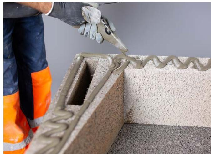
Apply the lip glue adhesive on top of the first layer.
