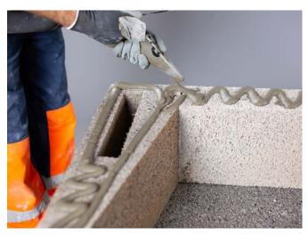
Apply the lip glue adhesive on top of the first layer.
