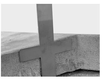
When the capping is being glued into place, slide the wave legs into the lip glue joint (as per pic).
