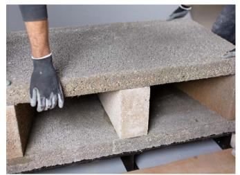
Press the base plate of the firechest down on to the log store. Keep checking all is level and remove any excess lip glue.
