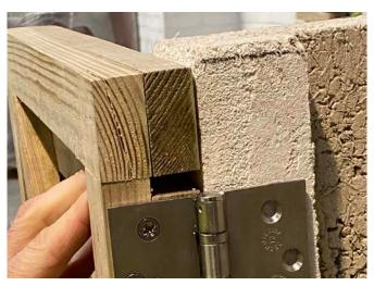
After rendering, align the hinge to the logstore, ensuring the door is below the top of the logstore (a 5mm gap is fine).
