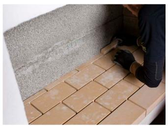
Complete the bottom layer of firebricks, then fasten the rear firebricks in place using the firebrick mortar. Use a tile spacer to keep an 8mm gap.
