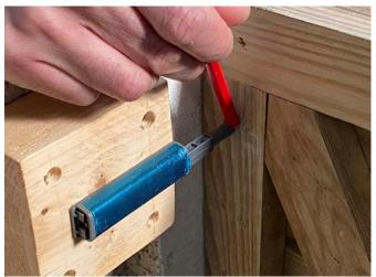
Mark with a pencil the end of the magnetic latch on the door.
