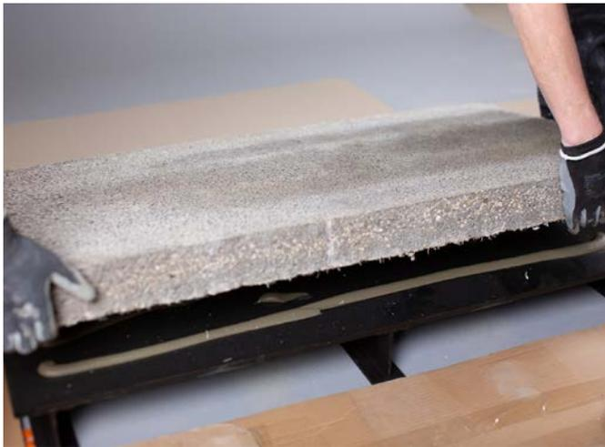
Create a suitable base. We recommend 100mm thick reinforced concrete. Bed the base plate using the supplied adhesive or mortar mix. Check every stage is level.
