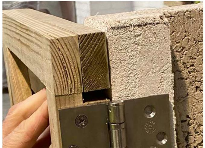
After rendering, align the hinge to the logstore, ensuring the door is below the top of the logstore (a 5mm gap is fine).
