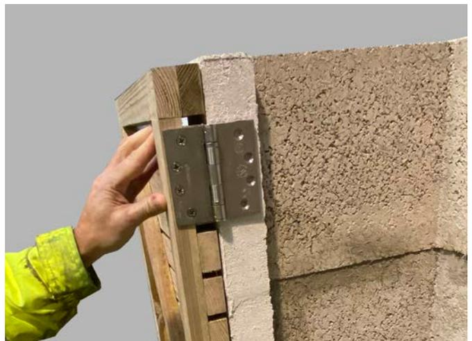
Secure the hinge to the pumice logstore with the screws provided.
